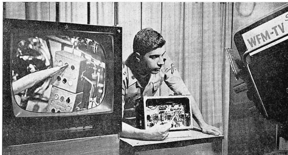
FIG. 31. An instructor points out small parts of electrical equipment as camera sends it out over closed-circuit TV. Monitor at left shows the result. Thus, students in classroom get excellent view of subject.
