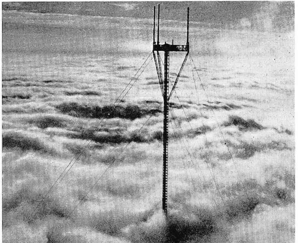
FIG. 10. The 1500-foot height of the candelabra often rises above a fog bank in the valley as shown in this dramatic photograph. The single structure, in spite of its height, is less of an air-traffic hazard than would be three separate towers.
