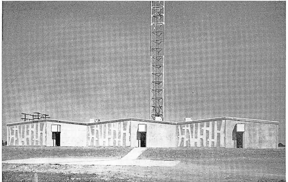
FIG. 2. Stations KCRA, KOVR and KXTV occupy essentially identical sections of the 3-section transmitter building. The base of the tower rests nearby to minimize horizontal transmission-line runs. The transmitter facilities of KOVR are in the section at left, KCRA in the center, KXTV in the right.
